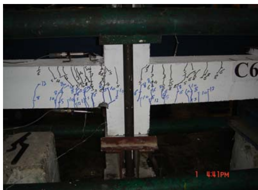
Fig. 4: Cracks pattern of test Specimen C6
